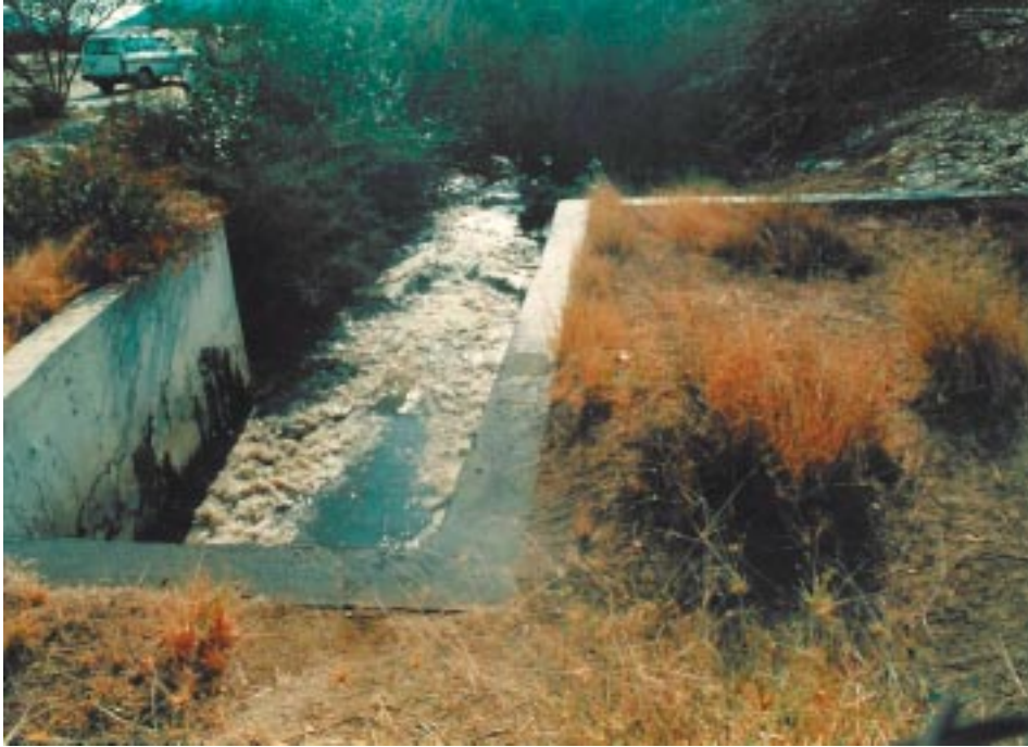
FIG. 1. Photograph showing the main outlet of the wastewater disposal to an open stream at Wadi Uranah.
